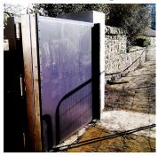
This impressive structure is part of the two giant floodgate sets recently installed on Warriston Road. Reader Neale Gilhooley photographed them, and has been told by the Council that they are required in case water is pushed over the riverside wall due to new, higher defences on the opposite bank.
