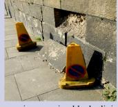
The seeming massive blocks lining the **embankment on Bellevue** are not as massive as first imagined, and some of the **facing stones** are now parting company from the **crumbly sandstone behind**. CEC is aware.
