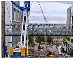
Installed in 2003 as part of the Omni Centre development, the 50m 'complex composite beam' weighed 90 tons and, because its foundations were divided by a geological fault line, was designed to move +/-15mm. If all its circular hollow tubes were straightened out and placed end to end on the road, we estimate they would stretch from their original site nearly to the junction of Inverleith Row and Terrace.
