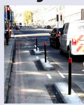
Cycleway delineators, known as 'kerb splitters' (short stretches of kerbs laid back-to-back, with collapsible/ reboundable bollards in-between) have been installed on Leith Walk at the junctions with Pilrig and Brunswick Sts. The previous unfit-for-purpose delineators ('orcas') were removed in a process which cycling correspondent Tim Smith terms 'orcastration'.
