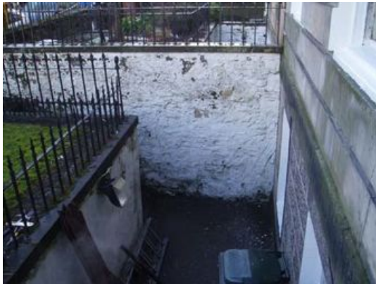
Figure 1: Lower ground boundary wall
