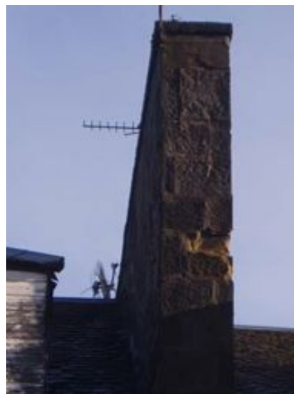
Figure 8 Rear right mutual chimney stack
