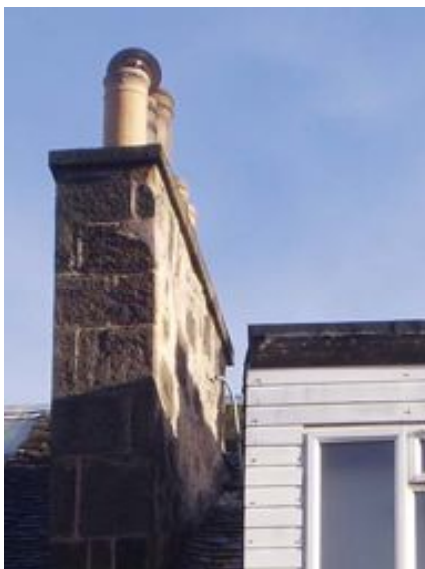
Figure 7 Rear left mutual chimney stack
