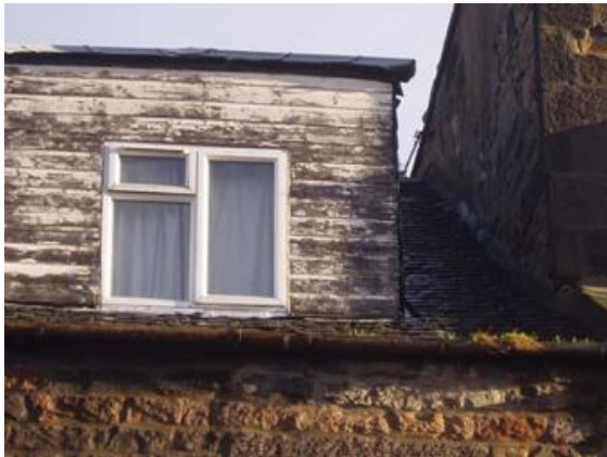
Figure 5 Rear right dormer and gutter
