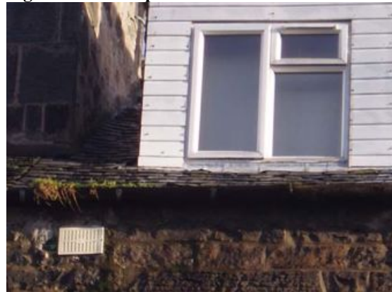
Figure 6 Rear left dormer and gutter
