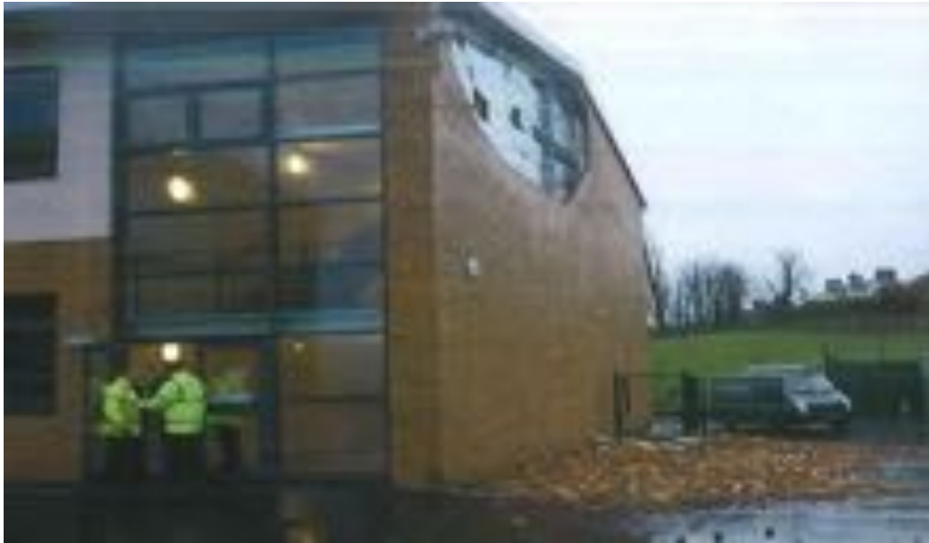
Image 26: Photograph of the collapsed panel at Trinity High School.
