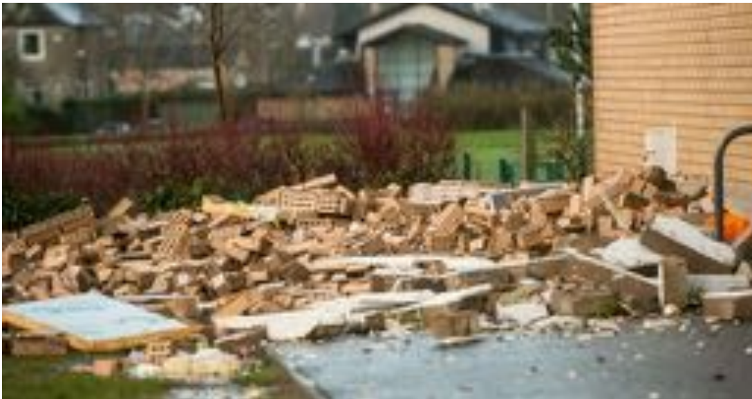
Image 3: Photograph taken at Oxfangs School of the gable wall after the collapse.
