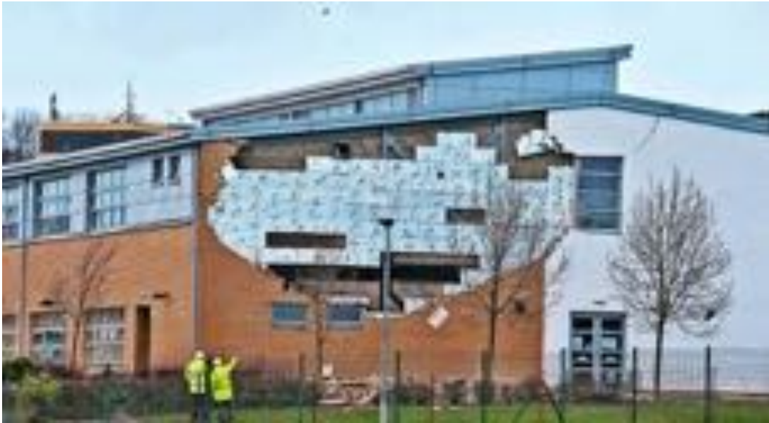
Image 2: Photograph taken at Oxfangs School of the gable wall after the collapse.
