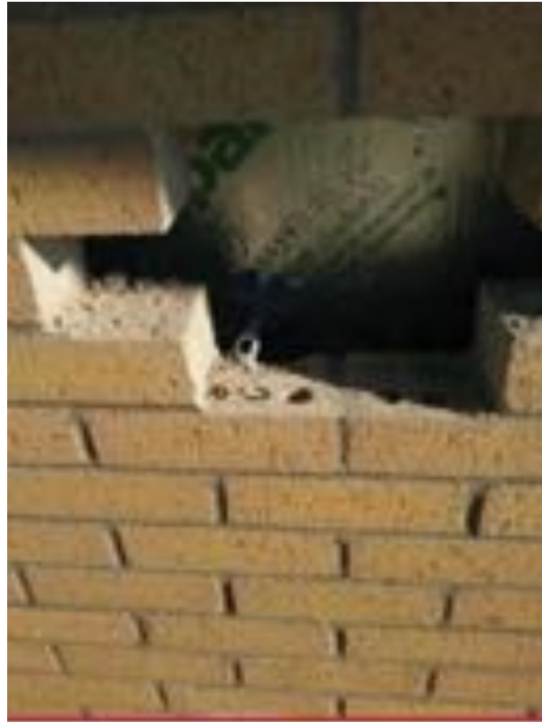
Photo 15.23.45 Location 40 – 35mm embedded
