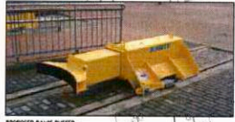
PROPOSED RAISED KERB BUFFER - TYPE 2 EB
